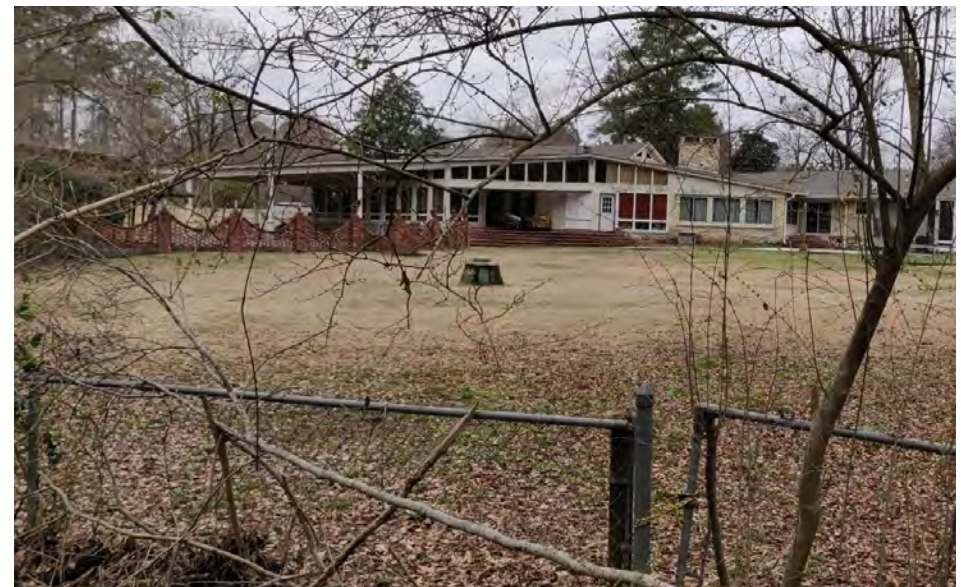
There are a few occurrences of private fences encroaching onto City of Birmingham land and the sewer easement. A full corridor survey is recommended to full assess the extent of these encroachments.
