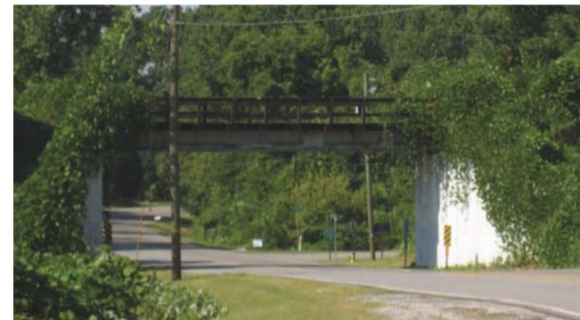
CSX Rail Bridge going over New Castle Road in Fultondale.
