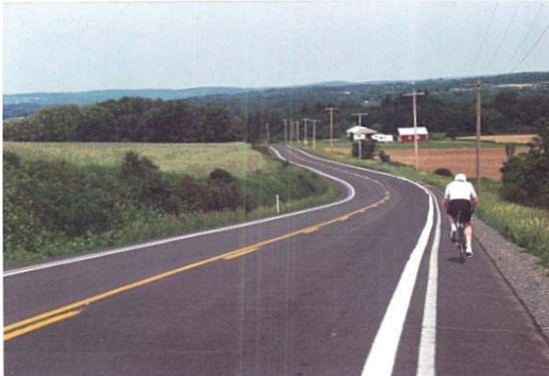
Providing paved shoulders on rural roads can improve safety for bicyclists, pedestrians and motorists.
