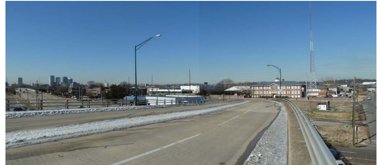
Figure 5.5 – 35th Street Bridge Trail
