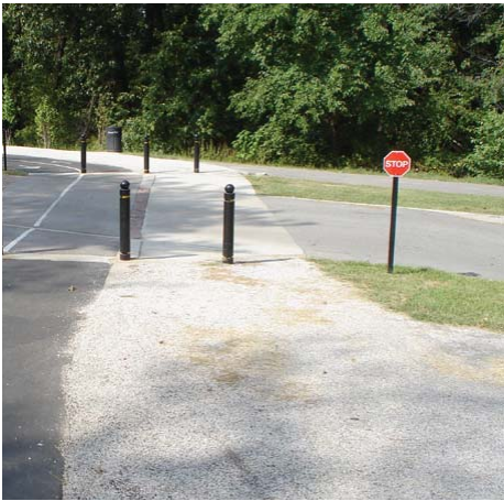
Bollards prevent motor vehicles from entering multi-use paths and trails, thus enhancing user safety.
