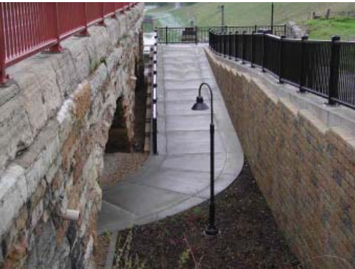
Adequate lighting increases trail safety.
